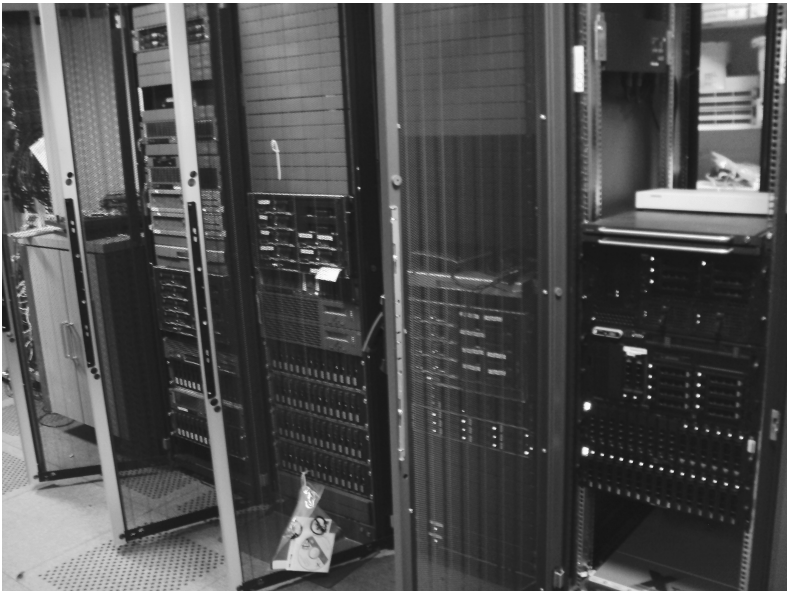
Fig. 2.1 Typical 2010's era radiology systems server racks with hard disk storage arrays. The server racks are housed in perforated metal cages to allow for high air-flow (for cooling).
