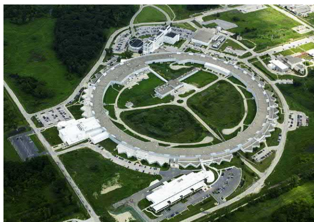
FIGURE 1.120 Aerial photograph of the Advanced Photon Source of the Argonne National Laboratory, Argonne, IL, USA, which houses a 1.1 km storage ring for the production and application of synchrotron radiation. For the color version of this figure, the reader is referred to the electronic version of the book. Courtesy of Advanced Photon Source, Argonne National Laboratory, Argonne, IL, USA; http://www.aps.anl.gov/ .
