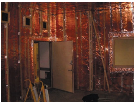
FIGURE 39-4. Copper RF shielding Faraday cage being built into an MRI room.
